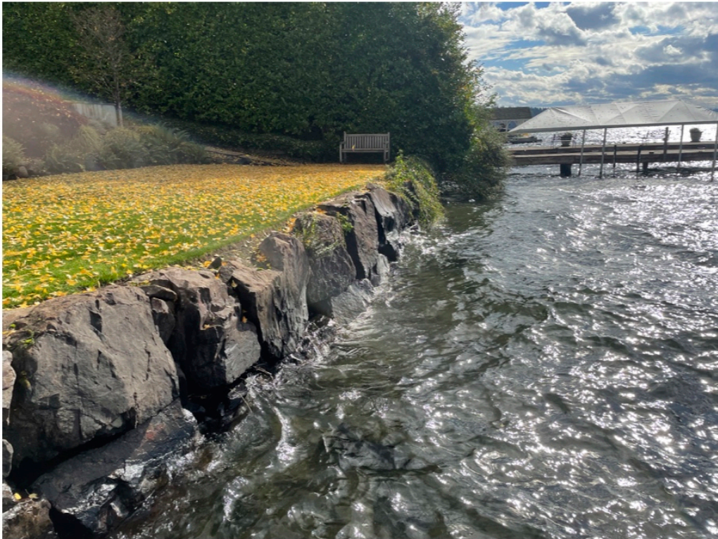
Photo 3 - Shoreline conditions looking south.
