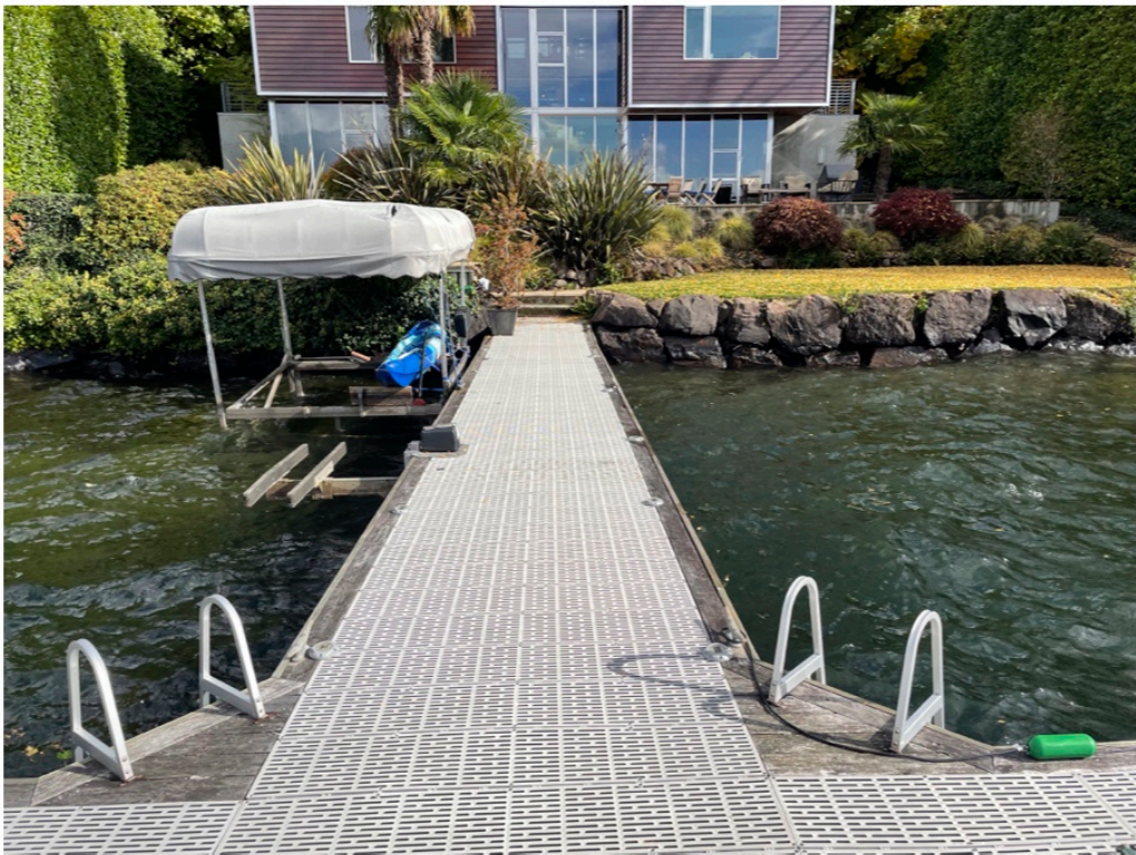
Photo 2 - Pier looking landward.
