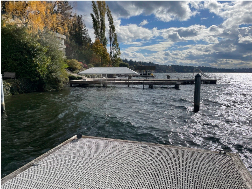
Photo 5 - Shoreline conditions south of property.
